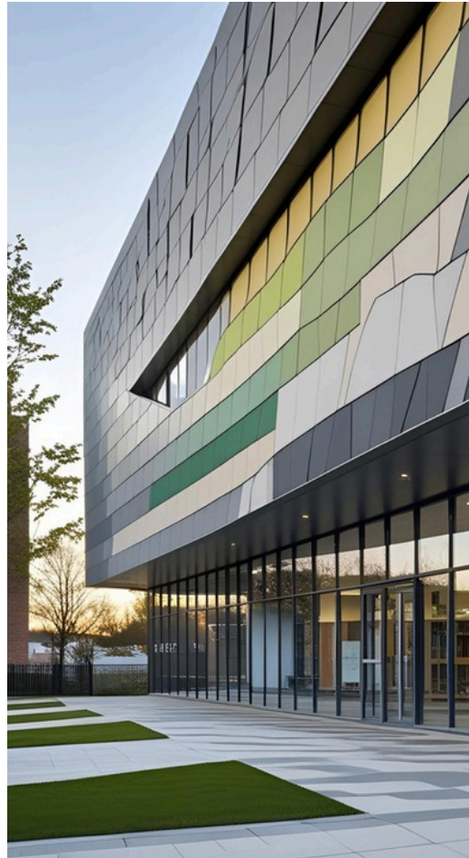
Public Library — Solid Colour Facade Cladding
